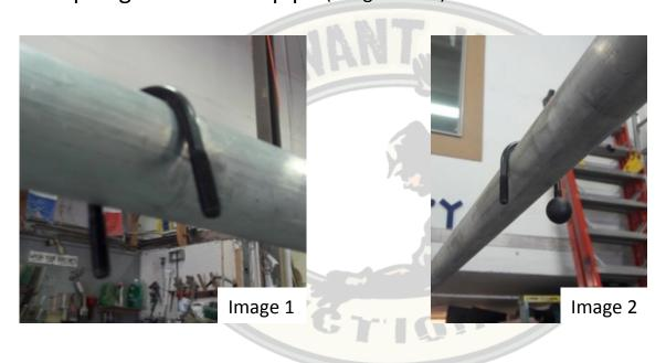
Step 2: Slide 2 Ends of Trim Chain Over the U Bolt creating a loop. Lock Down with The Ball End on the DS Side of the Pipe (Images 3 & 4)
