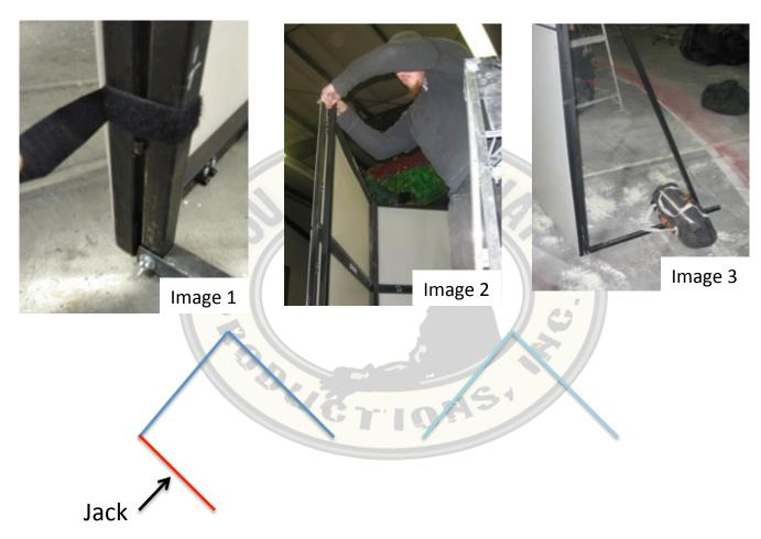
Step 3: Place a 50lbs Sandbag on the Back Edge of the Jack Base, Remove the Safety Rope from the stack and Open to a Flat Wall (Image 3)
