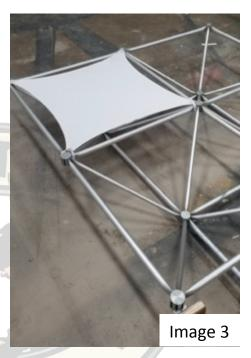
Step 3: Stand Unit Upright to pull the center of each Vortex back Use the Velcro or Ties and Attach directly to the Hub (Images 4 & 5)
